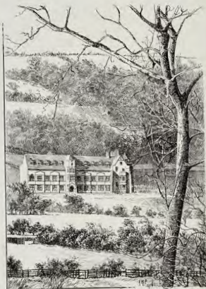
Ampleforth Preparatory School.
