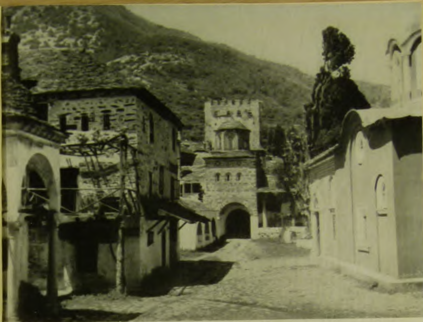
Mount Athos: the Meyisti Lavra: general view of the church and main buildings
