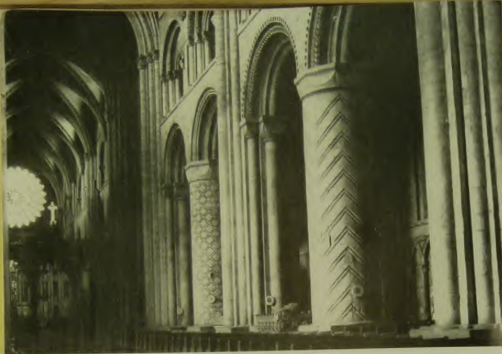
DURHAM CATHEDRAL The Nave pillars
