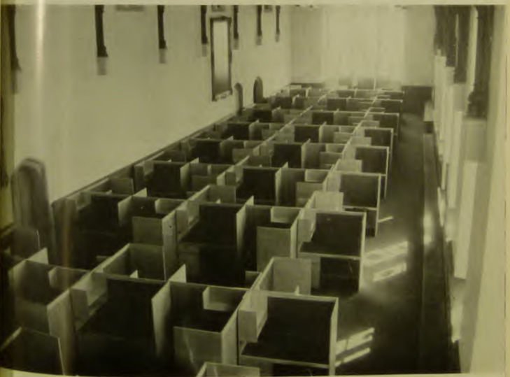
THE BIG STUDY WITH CARRELS, BEFORE THE NEW GRUCHEUX WAS INSTALLED
