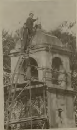
The Clock Tower under repair and renovation.
