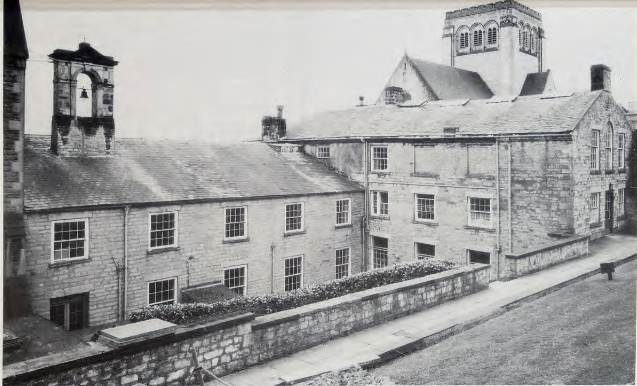
Bell Passage and the 1812 extension from the North. Notice the horizontal strengthening support on the East wall of the old dormitory above the monastery refectory which is referred to in Bede's Prest's letter, reprinted on page 7.
